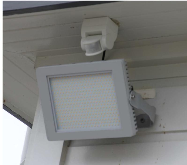
Floodlights consume a disproportionate amount of power and in some schools, run all night. On the left is a typical floodlight before replacement, - this unit burns through 400 watts of power every hour.
