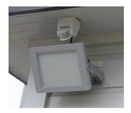
Floodlights consume a disproportionate amount of power and in some schools, run all night. On the left is a typical floodlight before replacement, this unit burns through 400 watts of power every hour.
